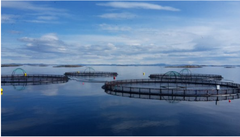
(a) Example of round fish pens. The round fish pens are the most common ones and are usually made of flexible material to make them more robust against a rough sea environment. To the bottom right, the locker described in section 3.1 can be seen.
