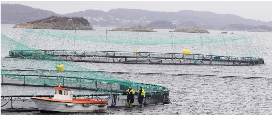
Figure 1.9: The superstructure of two circular plastic collar fish farms in the Bergen (Norway) area with two workers along the footbridge. (Heiko Junge, Scanpix)
