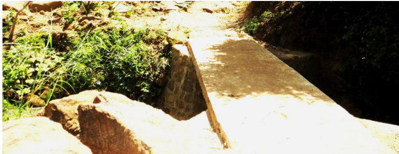
Photo 1. One of the two footbridges constructed. Source: Author
