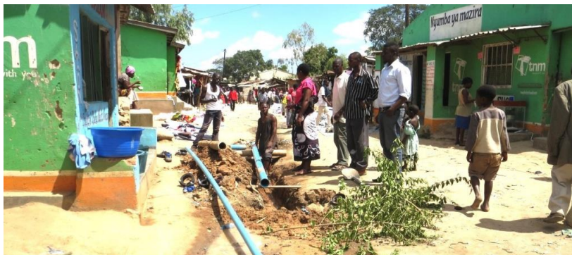
Photo 4. Workers from BWB fixing the water pipes. Source: Author
