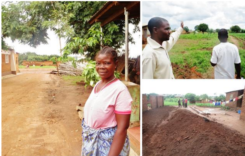
Photo 8. Left: Mrs Kawundu is one of the house owners who gave up a 1.5-metre-wide stretch of land along her house for this road. Upper right: Federation leader Mr Banda showing one of the planned roads. Lower right: A road that is being worked on by the church and its neighbours: Source: Author. Permissions to print names granted.
