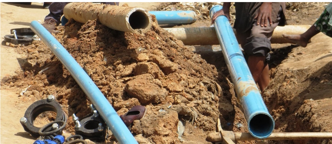
Photo: Workers from BWB fixing the breached pipe. Photo: Hilde Refstie
