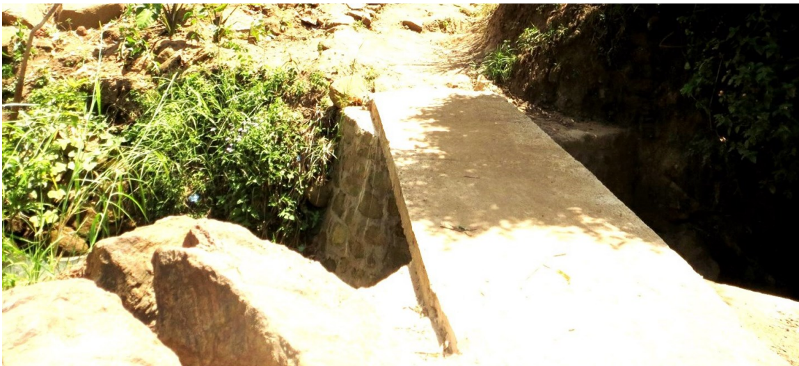
Photo: One of the three foot bridges constructed. Source: Hilde Refstie
