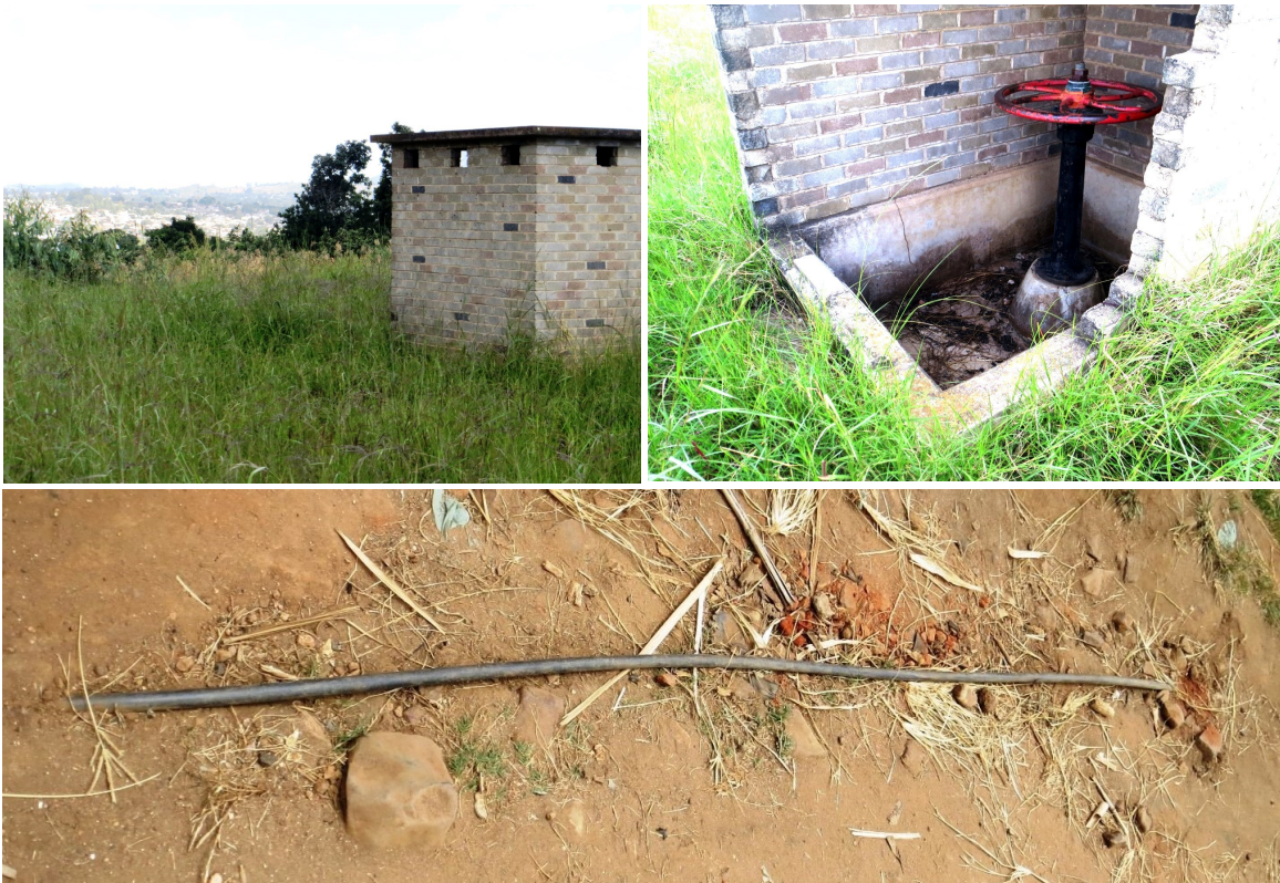
Photo: Upper section: Main water pipe house. Lower section: Pipe on road surface. Source: Hilde Refstie
