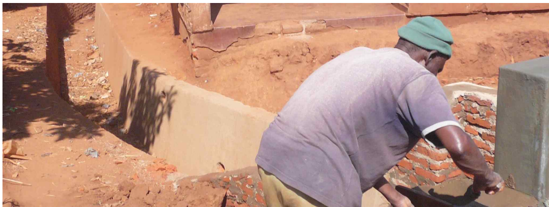
Building of drains in Chinsapo. Photo: Hilde Refstie
