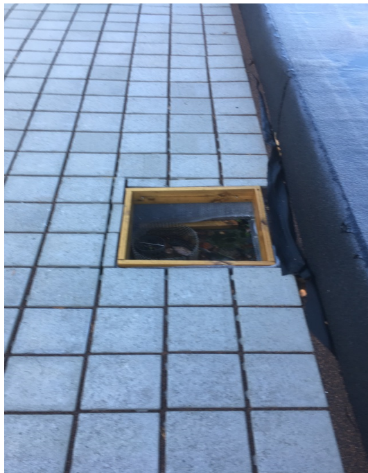
Figure 14: Outlet of the blue-grey roof
