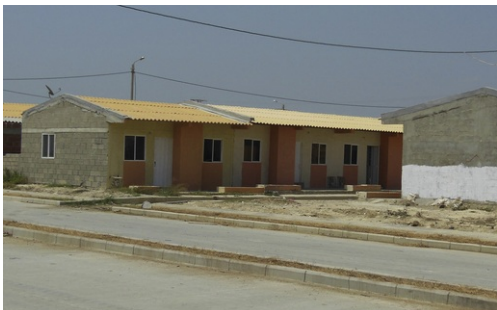
Fig. 3 Single-family row houses in VSP before occupation . Photo by the author.
