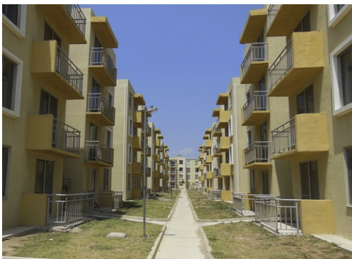
Fig. 4 Apartment blocks in VSP before occupation . Photo by the author.
