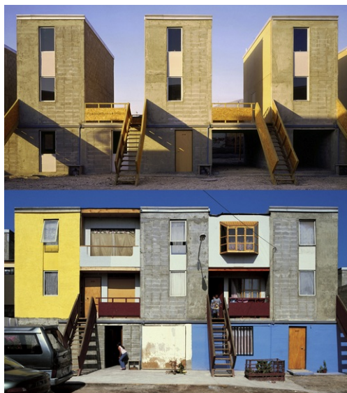
Fig. 11 Alejandro Aravena's incremental affordable housing units before occupation and a few years later. Source: Elemental chile.cl .
