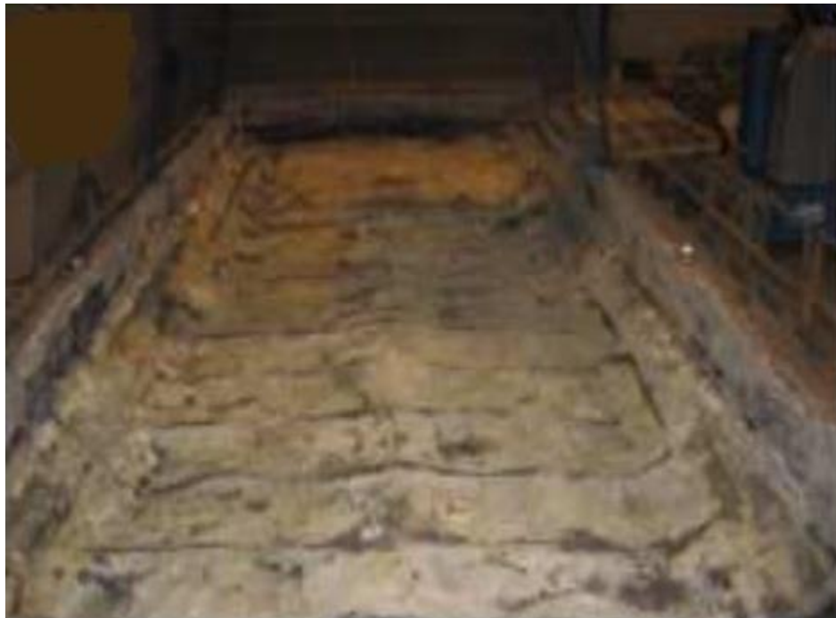
Figure 1.2. A worn cathode block after 5 years [4].
