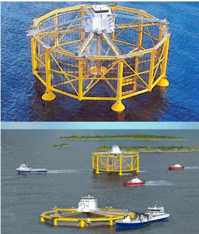
Figure 6. Salmar Oceanfarming platform in elevated and submerged conditions (Photos: Ocean Farming and SalMar, see also http://www.salmar.no/en/offshore-fish-farming-a-new-era ).
