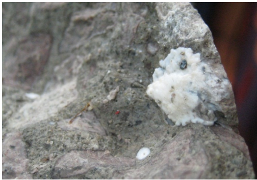
Figure 1. Alkali-silica gel present in an air void and in the interface between an aggregate particle and the cement paste in a concrete core drilled from a Norwegian dam structure.
