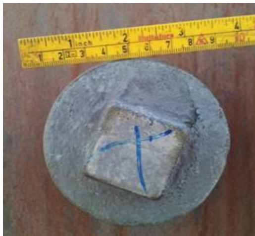
Fig..4.9: The diameter of the opening is around 9 cm.
