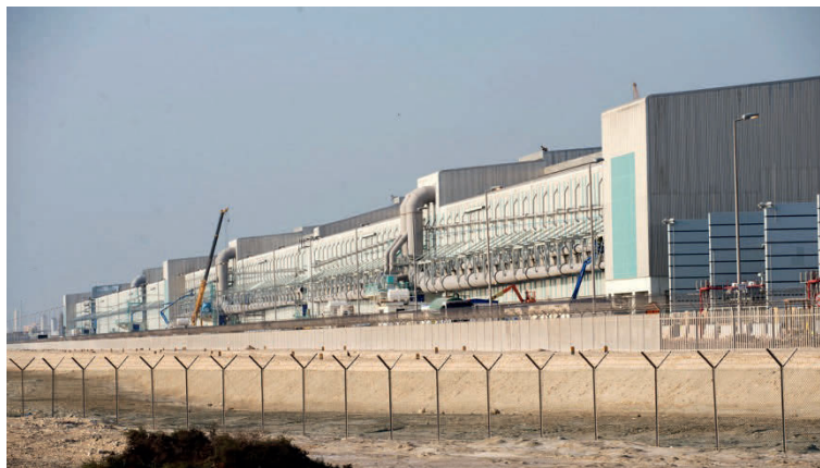
Figure 1.2: Image of a close to 1.2 km long pot room building at the Qatalum plant. Photo: H. Moland. © Norsk Hydro
