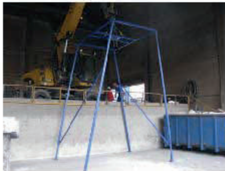
Figure 3. Steel frame for placement of the laser scanner.
