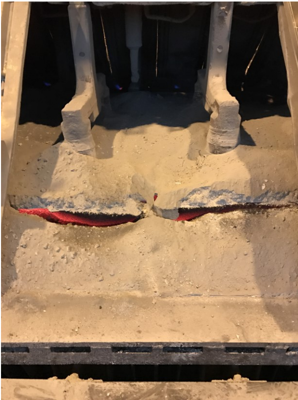
Fig. 1. Two anodes covered in mass, but with excessive tearing in front after long air-exposure. The front plate is shown in the bottom of the picture, and the current-leading yokes ascend from the mass, on top the anodes. Picture courtesy of Alcoa Mosjøen.
