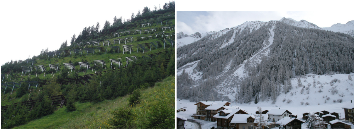
Figure 1.2: Protection forest support in effort to limit avalanche initiating within the trigger zone. Fences such as this are installed to enhance forest ecology through avalanche prone terrain. (Schild, 2006), (Jan, 2010)
