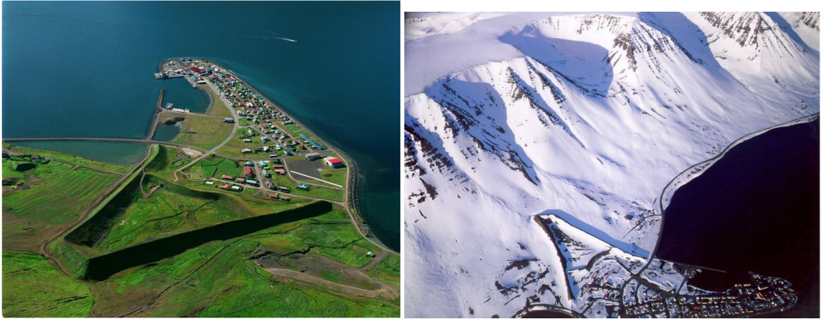
Figure 1.3: Conical earth mounds forming a barricade around Flateyri, a fishing vilage in the north-west of Iceland that suffered from a tragic avalanche event in October 1995 that resulted in twenty fatalities.
