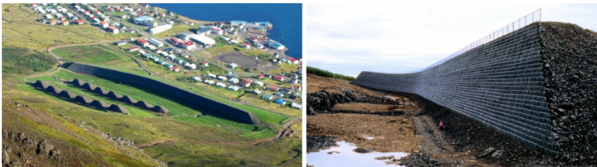
Figure 1.4: In 1974, Neskaupstadur damaged by a catastrophic avalanche so the settlement is now protected by a huge catching dam and cones. The maximum height is around 17 m. The photo shows the cones and catching dam below Drangagil. (Photo: The Icelandic Meteorological Office, IMO). Due to the height, most large dams in Iceland are made from "reinforcement material" on the impact side so that they can stand at a very steep angle.
