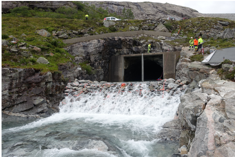
Figure 3.4.: Spillway outlet channel with a test dam covered with placed riprap (F15P2 in 2015). The crest of dam Svartevatn is visible in the upper right corner in the background. The discharge was provided from the reservoir impounded by the dam (Photo: NTNU).
