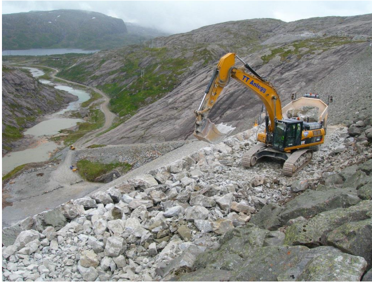
Fig. 1 Reconstruction of a placed single-layer riprap on the downstream slope of the 129 m high rockfill dam Svartevatn in Southwestern Norway. The riprap stones are placed one by one in an interlocking pattern and form with the adjacent filter layer an erosion protection against accidental leakage and overtopping. (Photo: NTNU)
