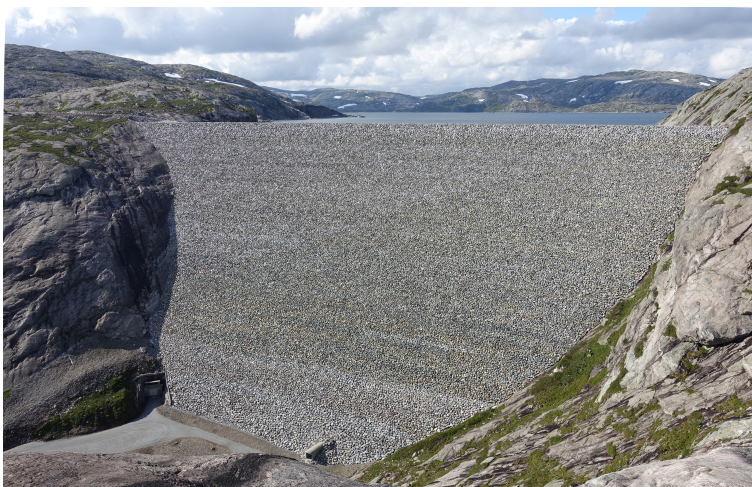
Figure 1.1.: Dam Svartevatn was with its height of 129 m the largest dam in Northern Europe when it was finished in 1976. The picture shows the dam after rehabilitation in 2015. The downstream slope is covered with placed riprap (Photo: P. H. Hiller).
