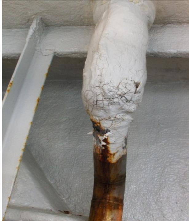
**Figure 3.4:** Picture of corrosion attack underneath insulation of pipe from an offshore platform in the North Sea.
