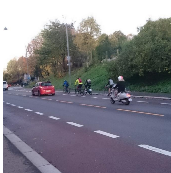
Figure 4: Bicycle lane in Oslo that is wide enough for two cyclists passing each other.
