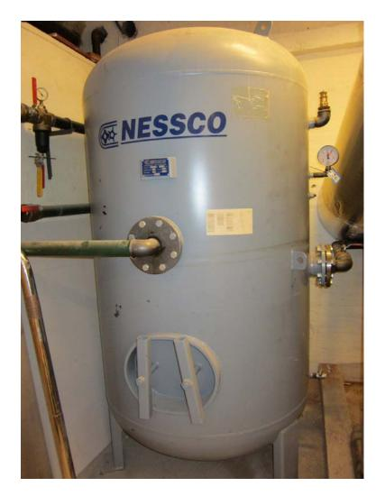
Figure 3.6: Air reservoir tank located in basement
