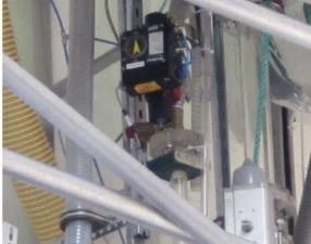
Figure 3.13: Choke valves; left: Fast valve, Right: Slow valve and its positioner
