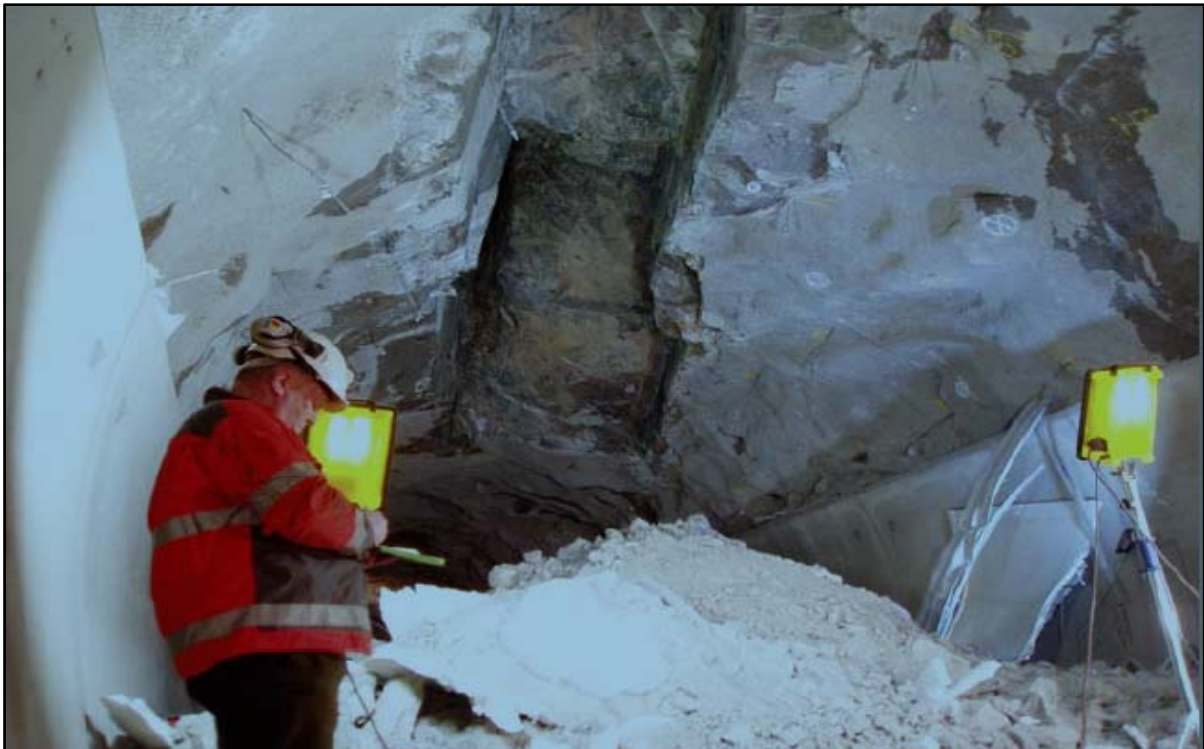
Figure 1. Photo of the collapsed area in the roof of the Hanekleiv tunnel and the material from the cave-in on the floor of the tunnel (Nilsen, 2012).
