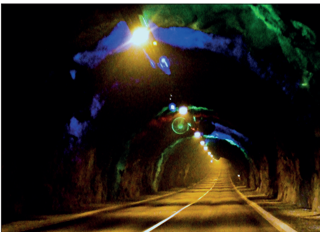
Figure 3. Norðoya tunnel was opened in 2006 (by Arne List (talk) – authors' own work, CC BY-SA 3.0, https://commons.wikimedia.org/w/index.php?curid=4233831 )
