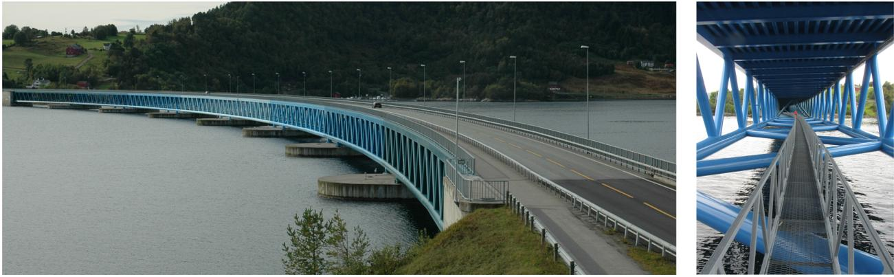
Figure 1: Left: The Bergsøysund Bridge viewed from the northeast end; right: the truss structure as viewed from below the bridge deck. Photo: K.A. Kvåle.
