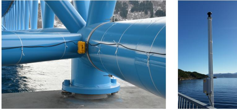
Figure 3: Left: accelerometer mounted on the truss; right: GNSS rover station at the middle of the bridge.
