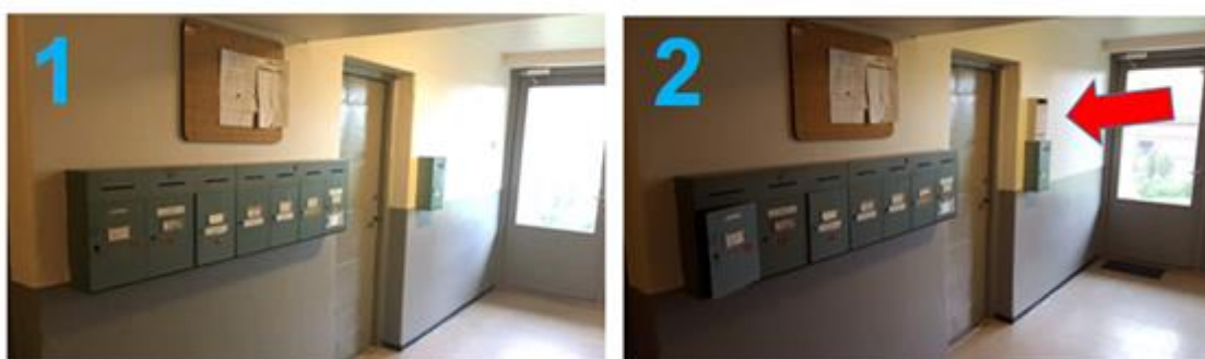
Figure 4.2: Hallway where the new mail box was installed. 1) Before mailbox is installed. 2) After mailbox is installed.
