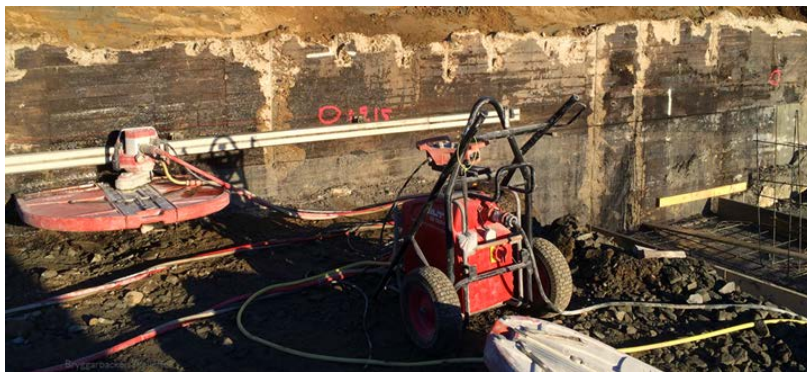
Figur 54 betongsaging vegger [31]
