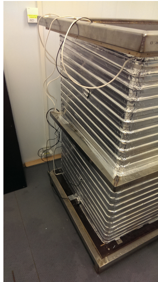
Figure 2.3: Heating cables on tank walls covered with aluminium tape, upper and lower section separated by the metal rod.
