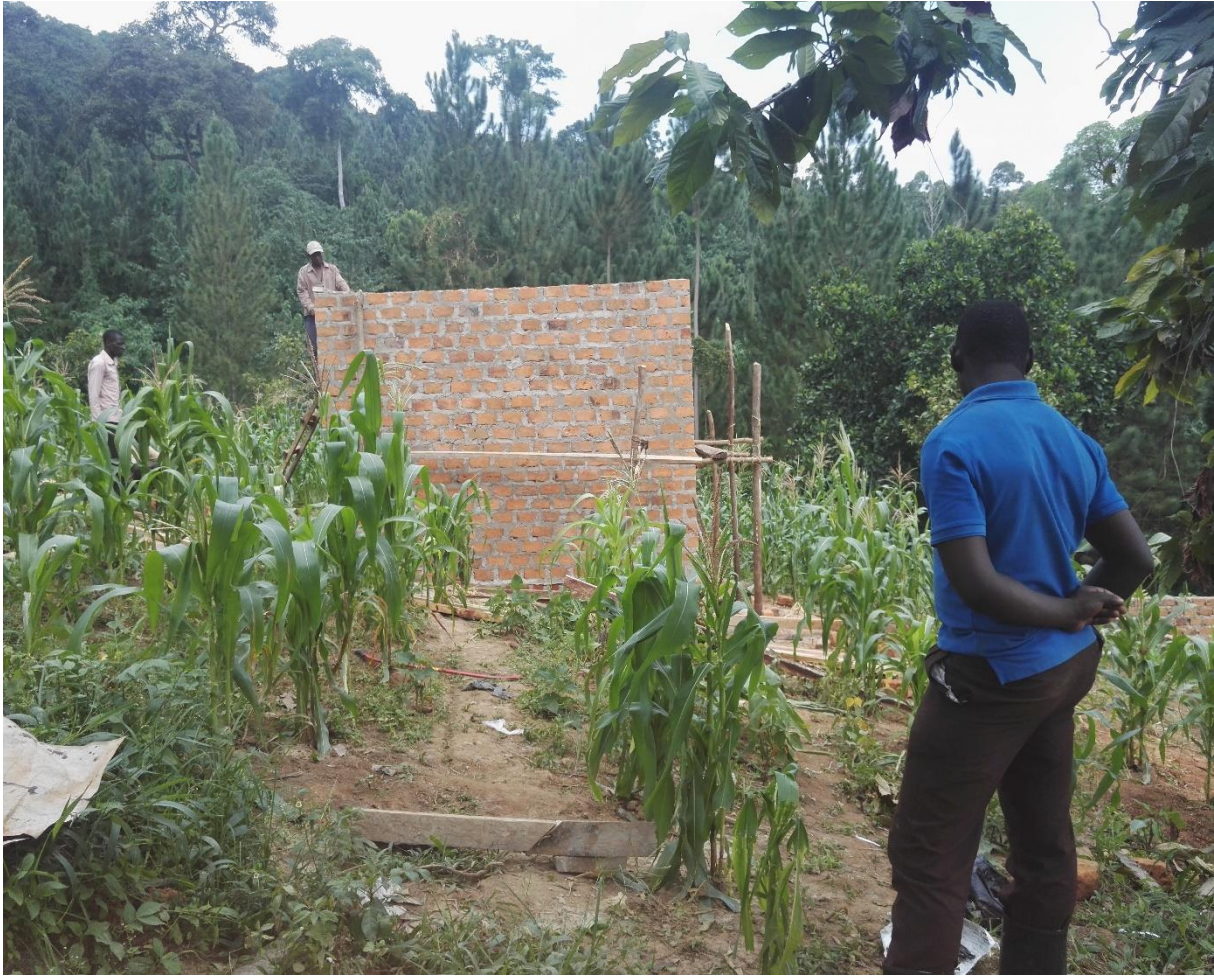
Figure 11 - Construction of a new house in Najjembe – private picture
