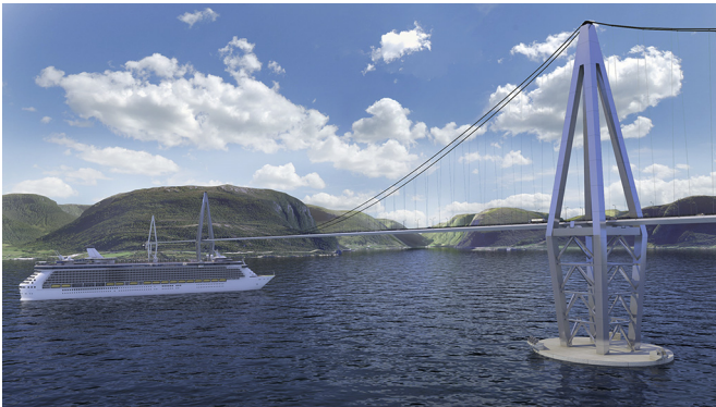
Fig. 2. Suspension bridge with floating towers, conceptual illustration (NPRA).
