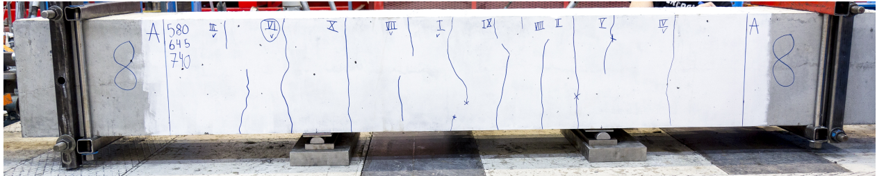
Figure E.15: Rissmønster for prisme 8- \phi 32-c40 for last 753 kN
