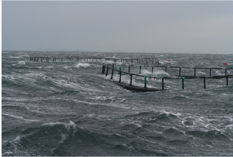
Figure 1: Illustrations of overtopping and out of water on the floater of a fish farm without net in a storm. (Photo: Marius Dahle Olsen)
