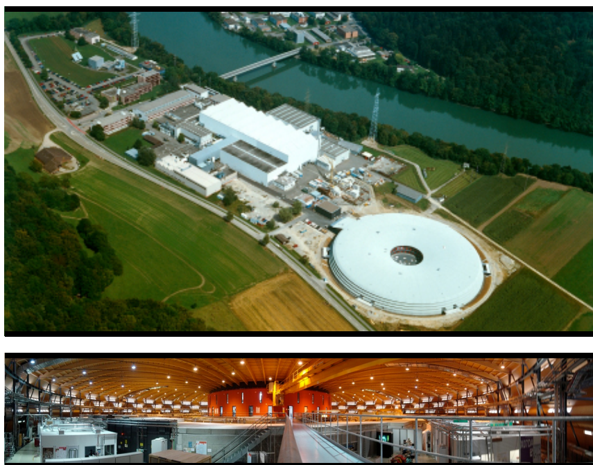
Figure 1.1: The Swiss Light Source synchrotron at the Paul Scherrer Institute in Switzerland is a third-generation synchrotron light source. With an energy of 2.4 GeV, it provides photon beams of high brightness for research in materials science, biology and chemistry. The circular building in the upper picture is the actual synchrotron. Inside there is an electron storage ring, 288 m in circumference, that provides electromagnetic radiation to more than a dozen beamlines.
