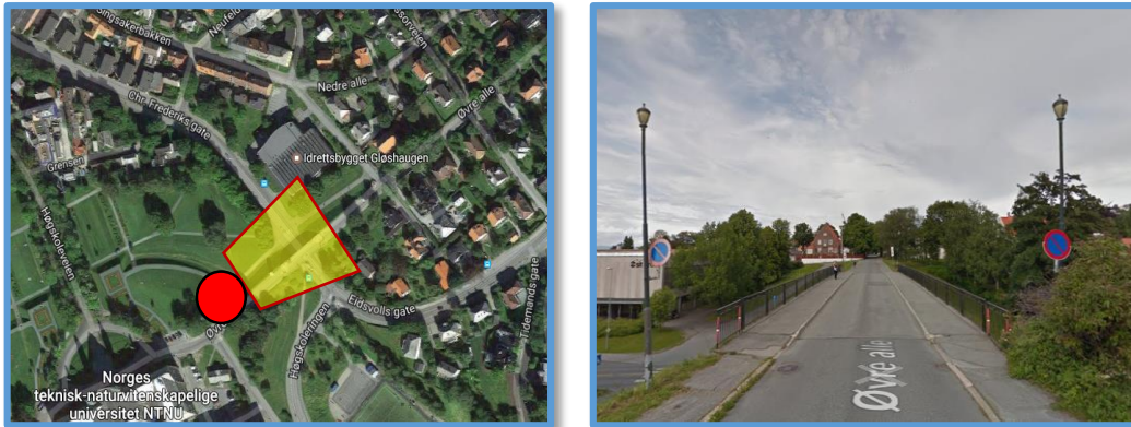
Figure 53 - Bridge over Eidsvolls Gate
