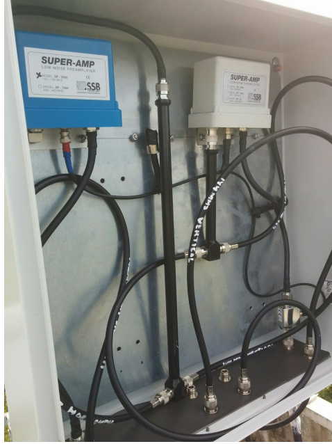
Figure 3.5.: Inside the LNA and phasing cabinet.
