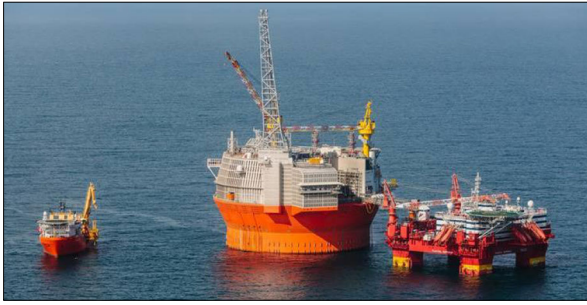
Fig. 12 The Goliat platform (photo by Eni 6 )
