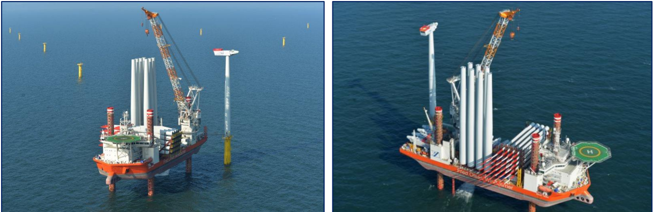
Figure 1.2 Existing OWT installations using jack up vessel [2]
