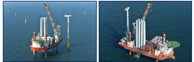
Fig. 2. Existing OWT installations using jack up vessel [2]
