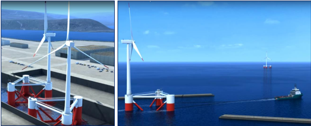
Figure 2.4 Onshore installation and towing of OWT [2]
