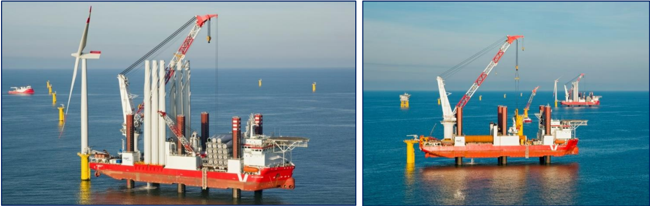
Figure 2.1 Installation of OWT using jack-up platform [5]
