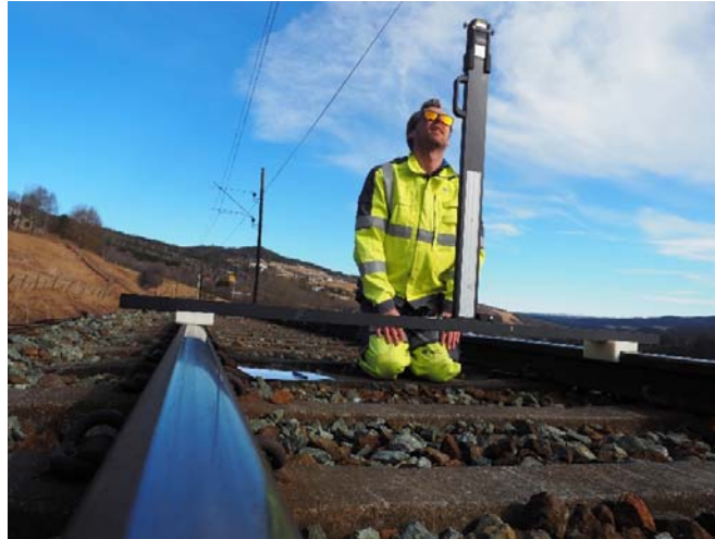
Figure 5. Measuring contact wire heights on site
