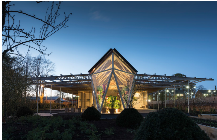
Figure 2: The roof structure of the Maggie's Centre in Manchester.
