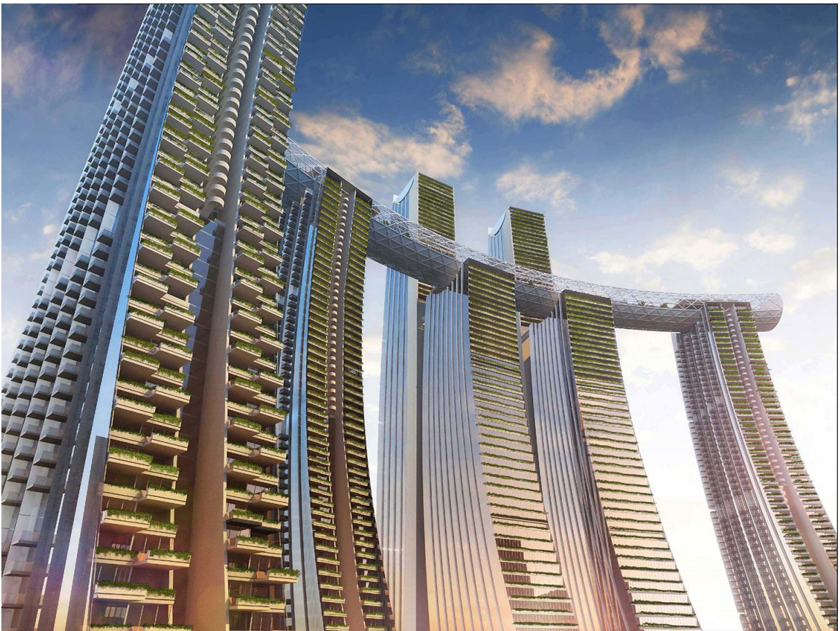
Figure 2.16 Raffles City in Chongqing. Photo from [p, 25].
