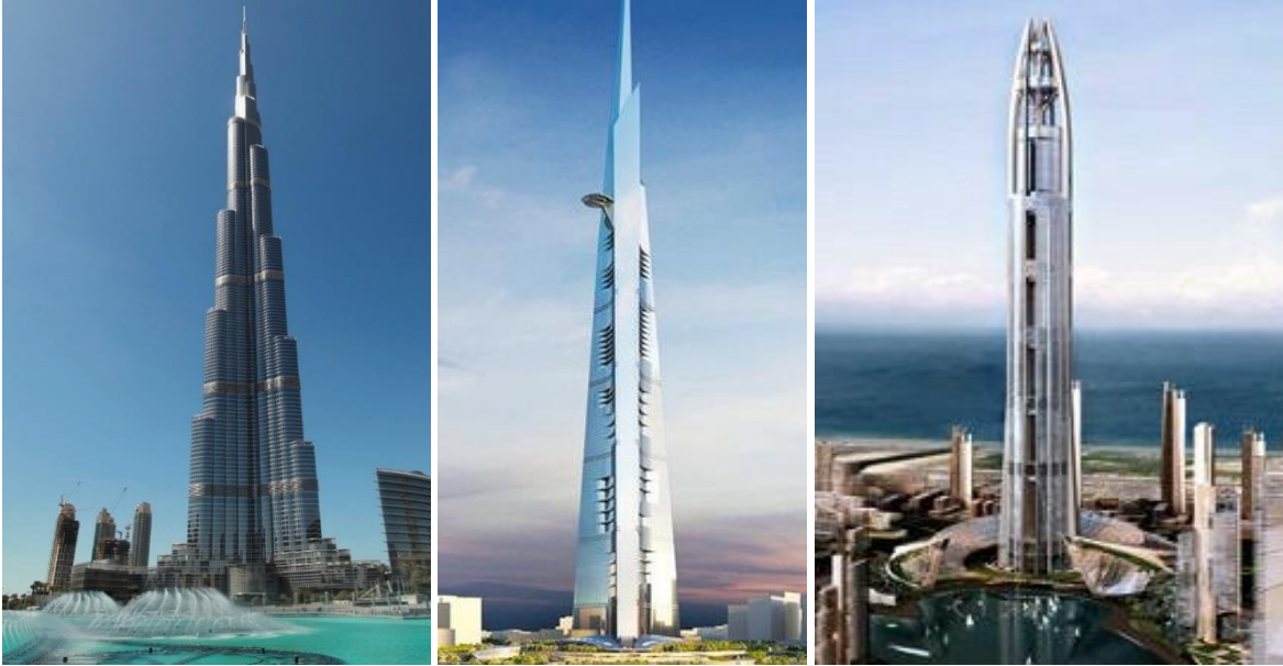
Figure 2.8 The Burj Khalifa (left), Jeddah Tower (center), and Nakheel Tower (right). Photos from [p, 14], [p, 15] and [p, 16].
