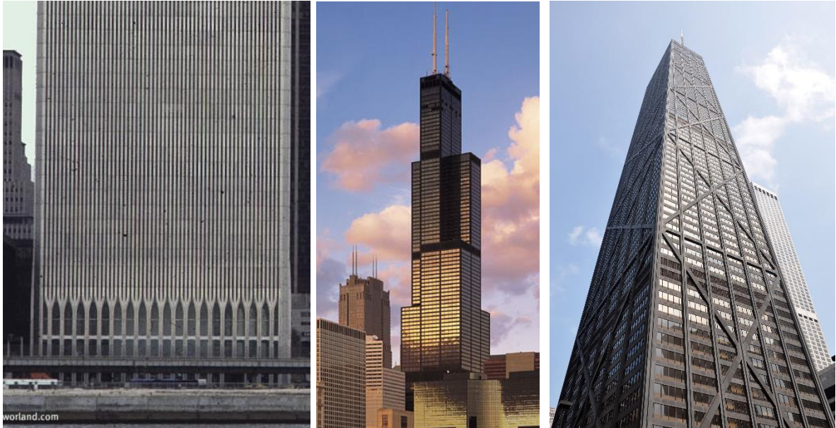
Figure 2.5 The bottom of a World Trade Center tower (left), Willis Tower (centre), and John Hancock Building (right). Note how closely spaced the columns in the World Trade Center tower area the bottom 2 floors. Photos from [p, 9], [p, 10] and [p, 11].
