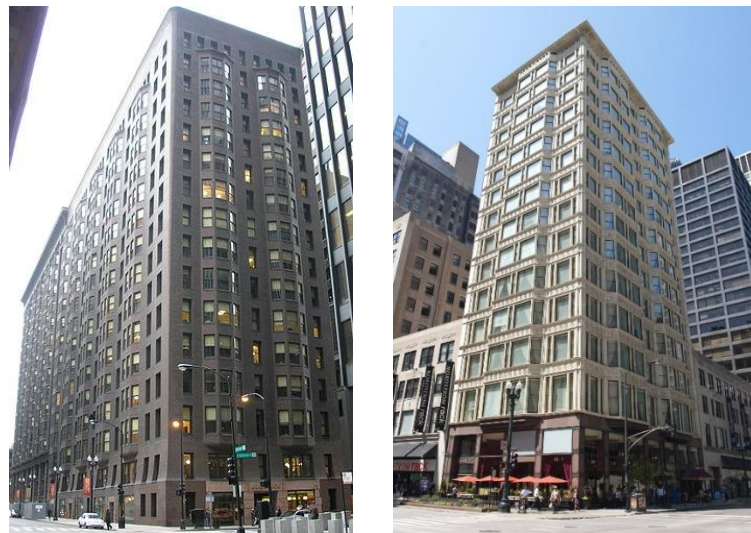
Figure 2.1 The Monadnock Building (left) and Reliance Building (right). Note the 2m thick bottom walls for the Monandnock building. Photos from [p, 2] and [p, 3].
