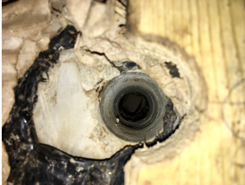
Figure 7.4.3: Picture of the drilled hole on the on-site test day
