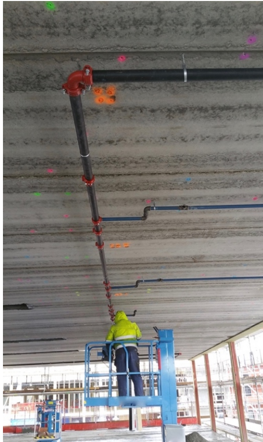
FIGURE 4.30 TEST OF INNER WALL PLACEMENT (OLE ROSENLUND, 2017)
