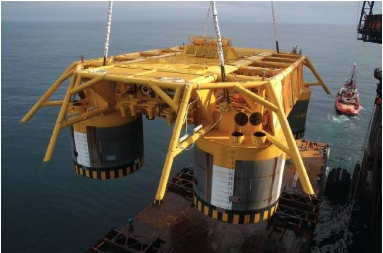
Figure 2.5: ITS being lowered of a barge. (Picture: Hydro)
