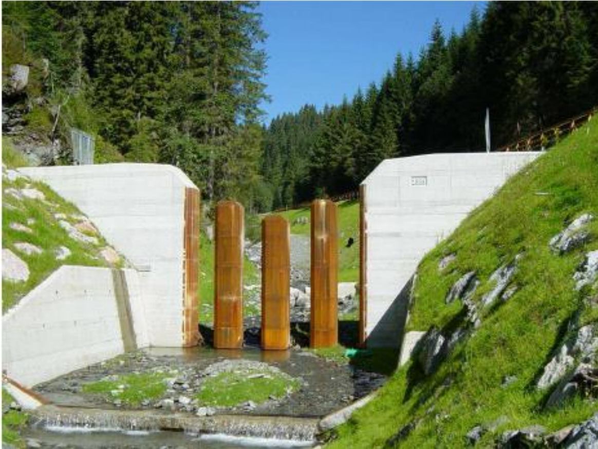
Figure 9. Schematic view of a debris flow breaker for energy dissipation (Rudolf-Miklau, Hübl, & Suda, 2014)
