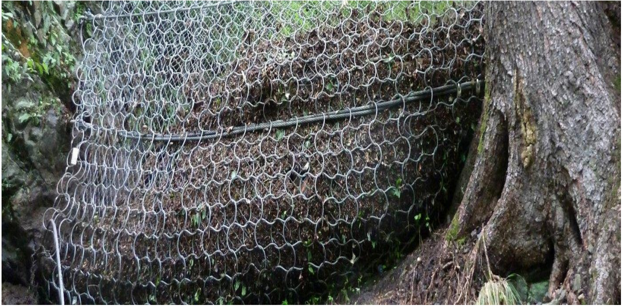
Figure 11. Wire net trapping debris (Mizuyama, 2008)
