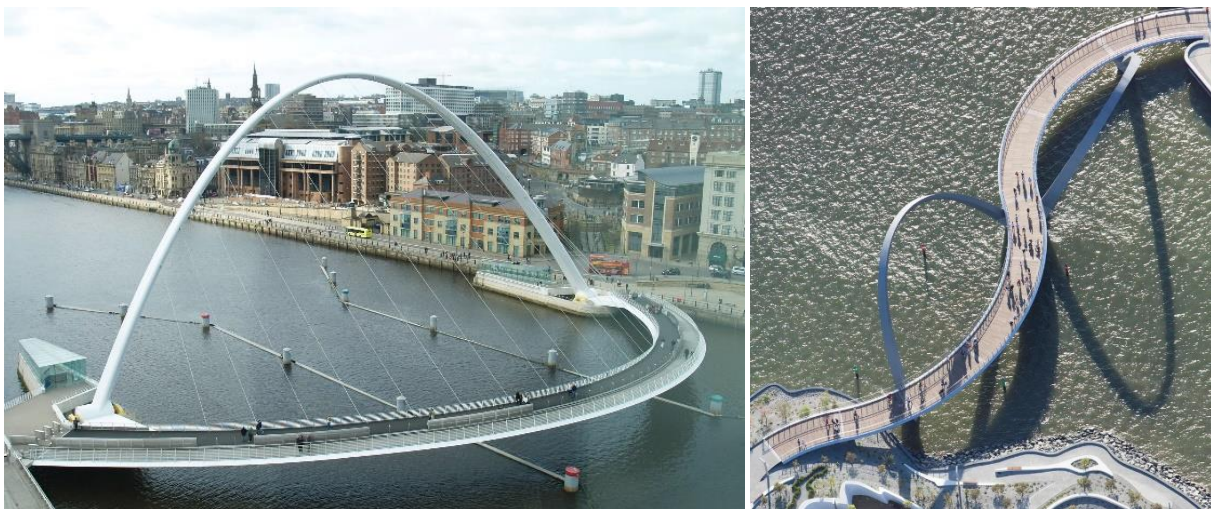
Figur 3.16. Venstre: Gateshead Millenium Bridge (Roberts, 2007). Høyre: Queen Elizabeth Quay Bridge (Jacaranda Photography, u.å.).
