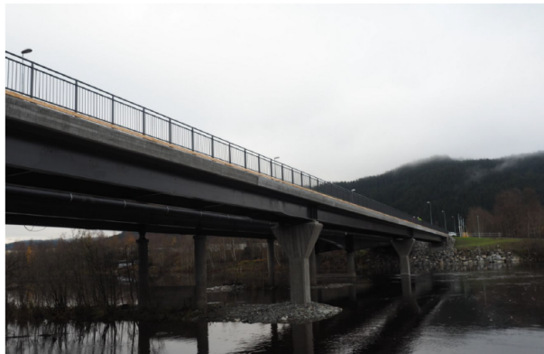
Figure 6.1: Picture of Bårdshaug Bridge [3]
