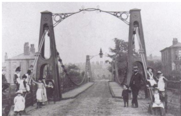
Figure 1.1: Broughton Suspension Bridge in 1883, rebuilt after the collapse in 1831
