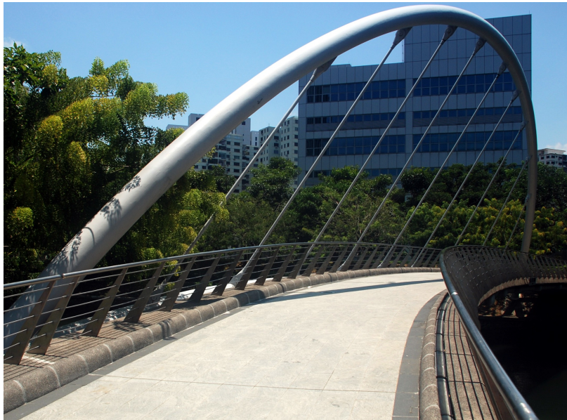
Figure 3.7: Jiak kim Bridge, vaguely longitudinal view. Photo credit: [6].
