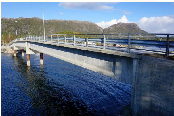
Figure 11.5: Bridge between Amundsøya and Brattøya
