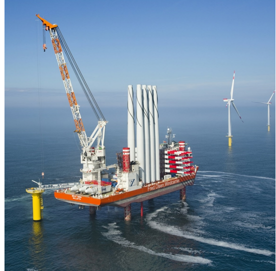
(b) Fred. Olsen Bold Tern lifts with configurations on deck for carrying nacelles, towers and blades (Fred. Olsen Windcarrier, 2016a)
