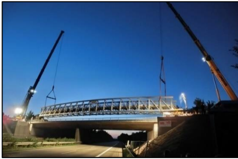
Figure 13: Aluminum pedestrian bridge assembled and installed over A5 in Germany [39].
