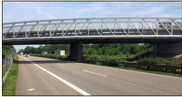
Figure 13: Aluminum pedestrian bridge assembled and installed over A5 in Germany [39].
