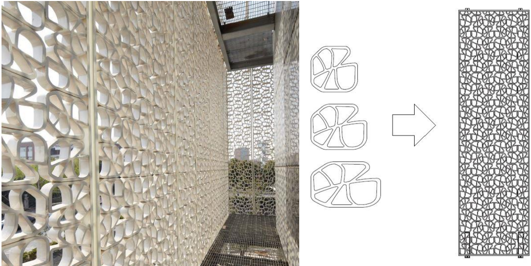
Figure 3-3: The two layers of the facade (left) and the external facade configuration (right) [56]
