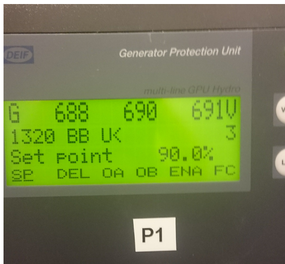
Figure E.1: U<< set point setting for DG1
