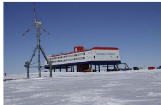
(b) Jacked up foundation in a building in Antarctica ( Neumayer Station III ) (from Tin et al. (2010))
