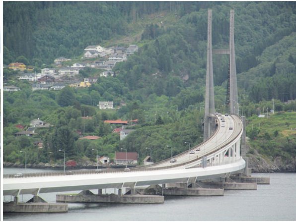
Figure 2.10: Nordhordalands Bridge (Underskog).
