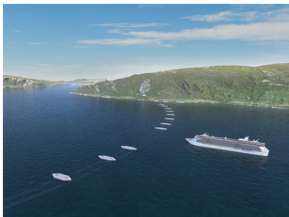
Figure 2.4: Pontoons on the surface of Sognefjord (Reinertsen and Dr. techn. Olav Olsen, 2013).
