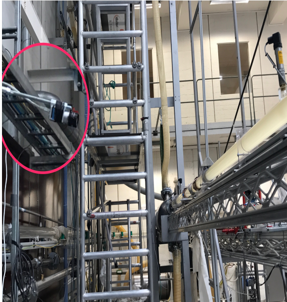
(a) Camera set up for horizontal pipe.
