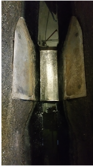
Figure 2.11: Drained Palmer-Bowlus flume at Risvollan [Photo PPN]
