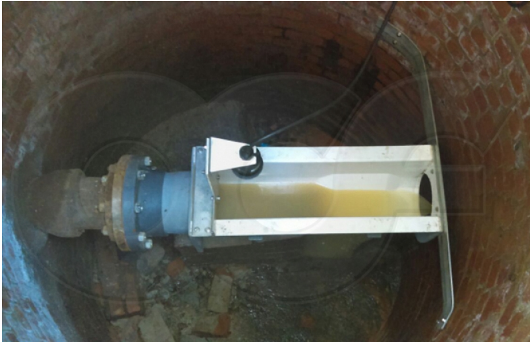
Figure 2.10: Prefabricated Palmer-Bowlus flume in operation from Open-Channel-Flow [8]
