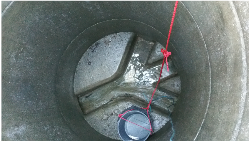
Figure 7.9: Piece of paper stuck in the bottom of a node
